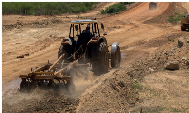
RETOMADAS AS OBRAS NA BR-226
