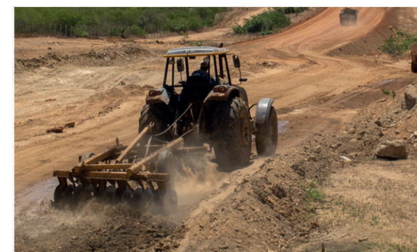
RETOMADAS AS OBRAS NA BR-226
